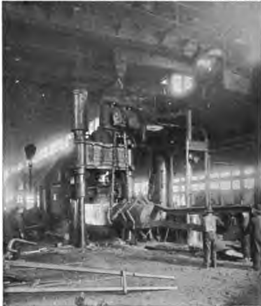
FIG. 240.—Hydraulic Press Forging Ingot.
